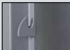
Main door latch hooks welded to frame
